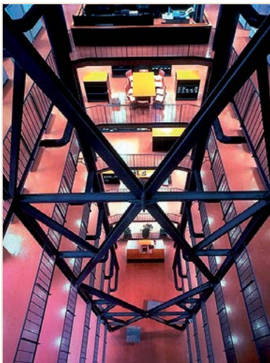
ArcelorMittal office building (AOB), Esch-sur-Alzette, Luxembourg
