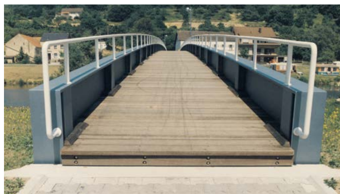
Footbridge in Steinheim, Germany
