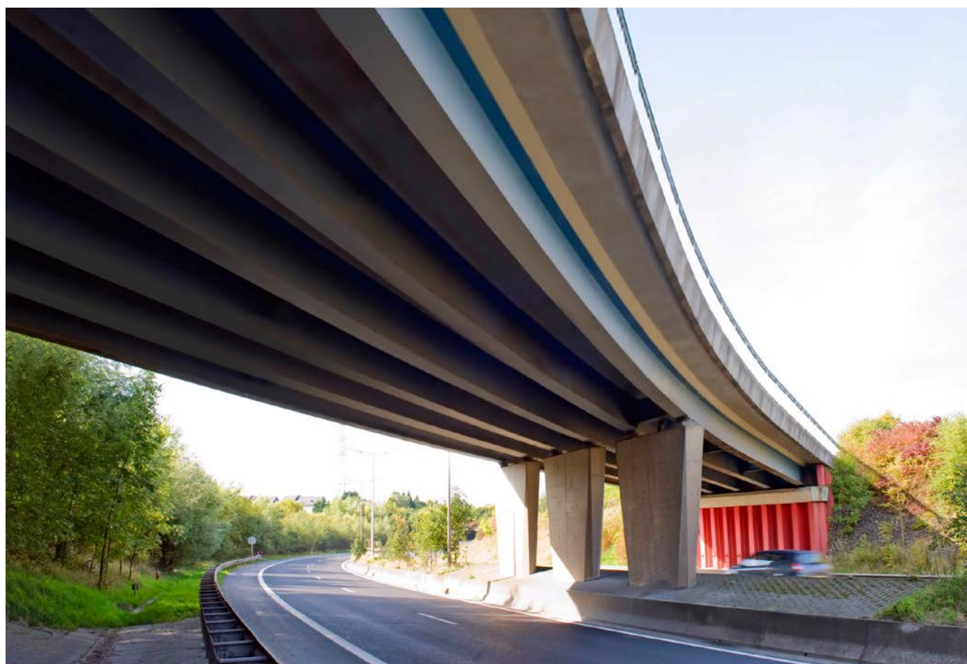
Multi-girders composite deck out of rolled sections, Soleuvre, Luxembourg
