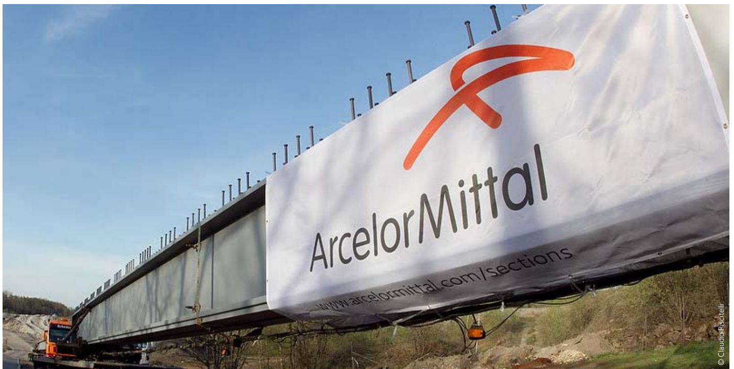
Delivery of a 41.7 m fully finished heavy section of a bridge on the B6N express way in Bernburg, Germany
