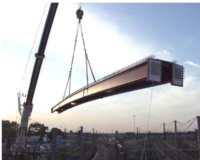
Choisy bridge, Villeneuve-Saint-Georges, France
