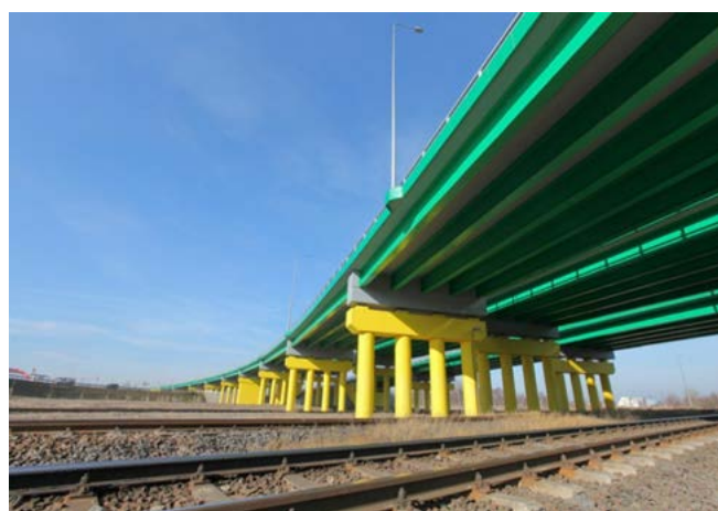
WD7 and WD8 viaducts, Gdansk, Poland
