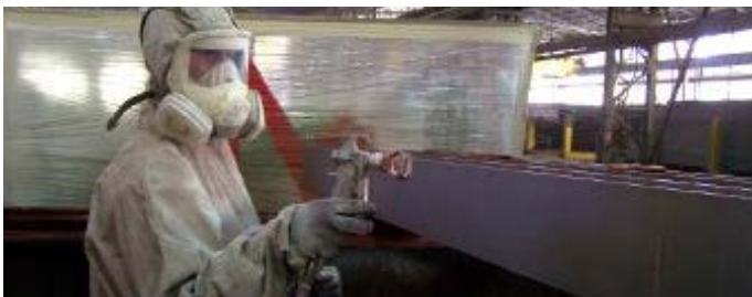
Manual application of an organic layer
