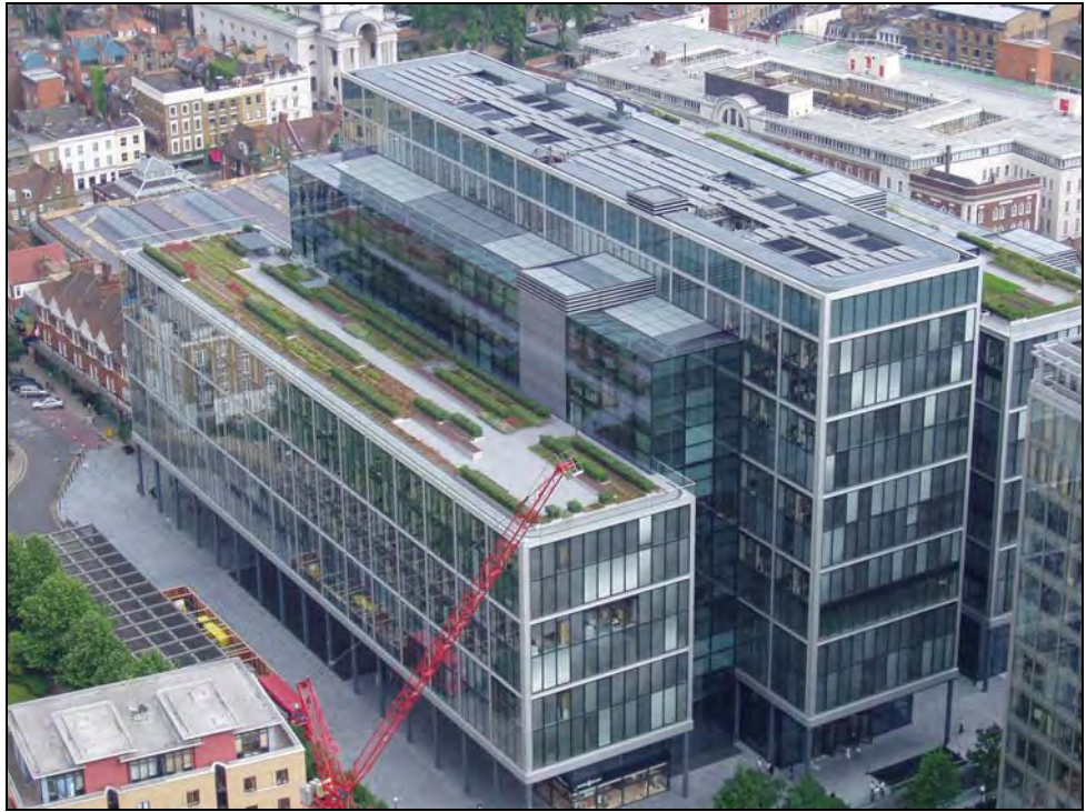
Figure 1.6 'Green' roof and PV panels attached to a city centre office building
