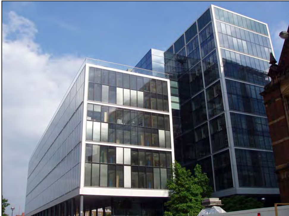
Figure 3.1 Office building, Bishop's Square, London
