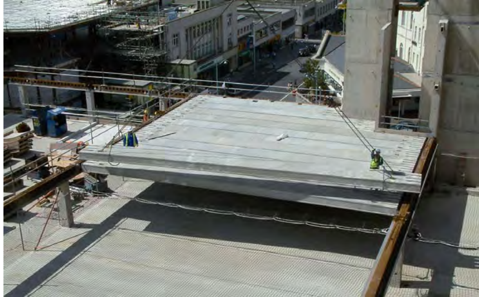
Figure 5.13 Long span precast concrete units being placed on steelwork
