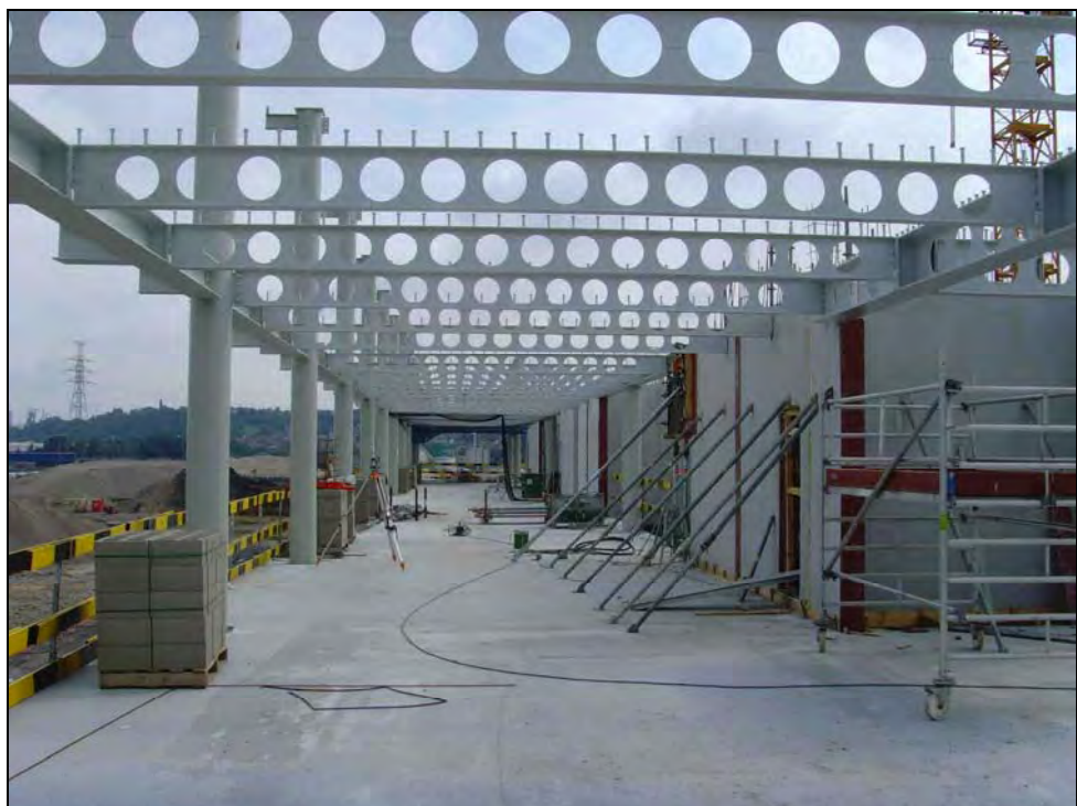
Figure 3.10 AM building during construction showing the cellular beams
